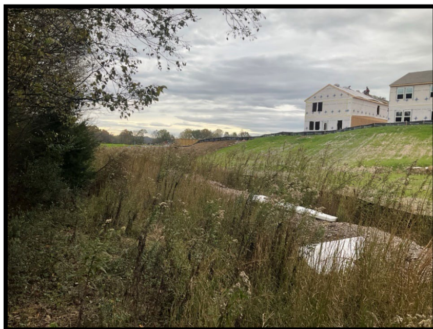
Photo 17 - View of the In/Near Stream Construction
