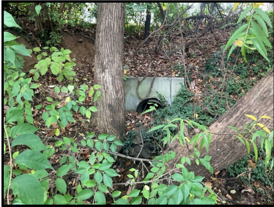
Photo 12 - View of the Pipe Outfall
