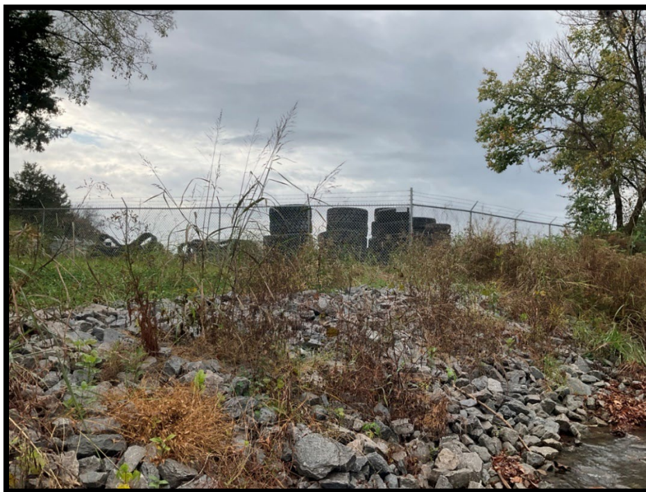
Photo 25 - View of the Inadequate Buffer
