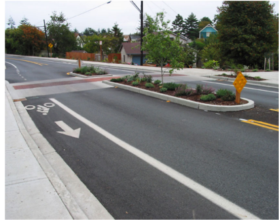
Raised medians reduce the width of the adjacent travel lanes.
