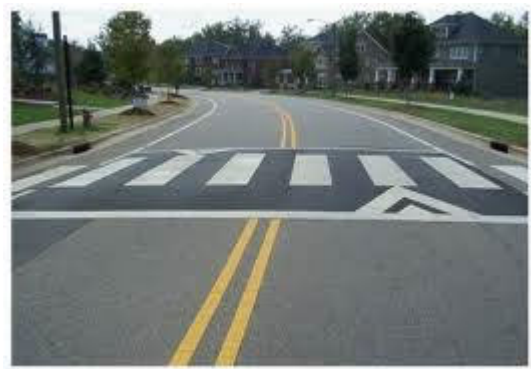
The speed table/hump that may be used in the City of La Vergne is 22 feet long and three inches in height.
