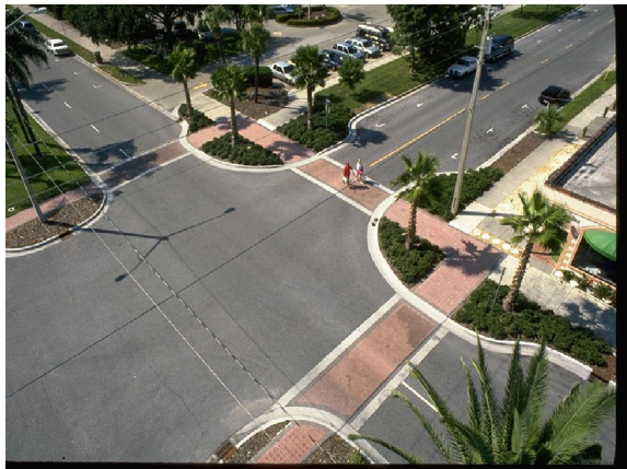
Curb extensions reduce the width of the roadway at intersections and create shorter crossing distances for pedestrians. The reduction in lane width encourages motorists to slow down when driving through the intersection.
