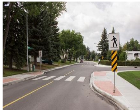
Curb extensions can be installed at mid-block locations to calm traffic in residential neighborhoods.
