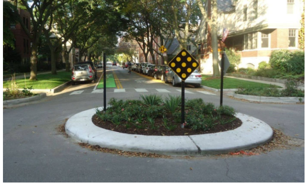
A traffic circle creates a horizontal deflection in the roadway, which causes motorists to slow down as they travel through the intersection.
