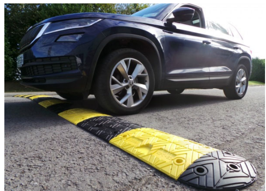
Speed bumps increase emergency response time for public safety vehicles and are associated with liability concerns.
