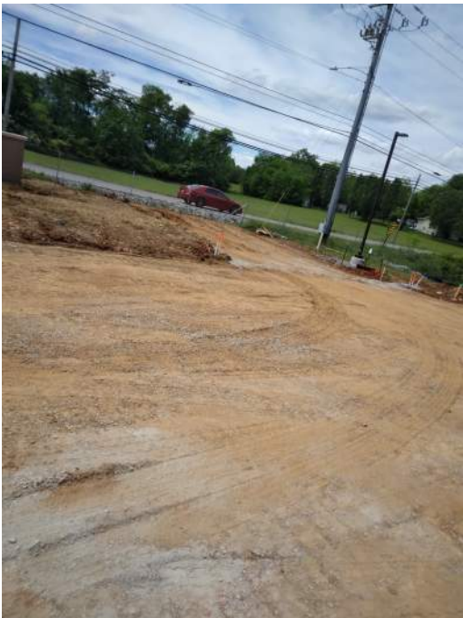
More of proofrolled area
