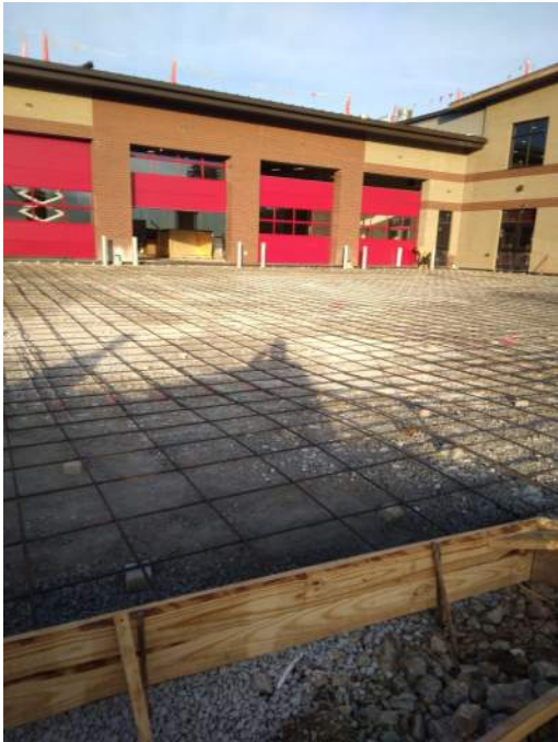
Rebar layout where concrete pour would occur
