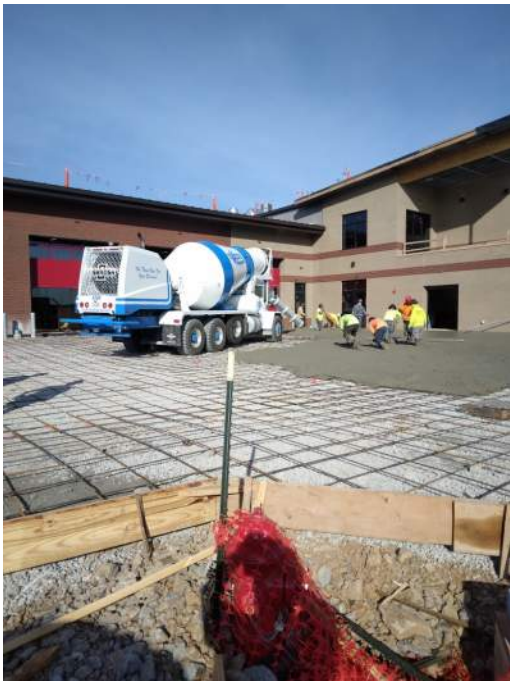
Pour location during application
