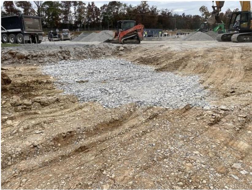
Description: View of previously placed stone Image Date Taken: 10/27/2023 Photographer: Hughes, Tyler
