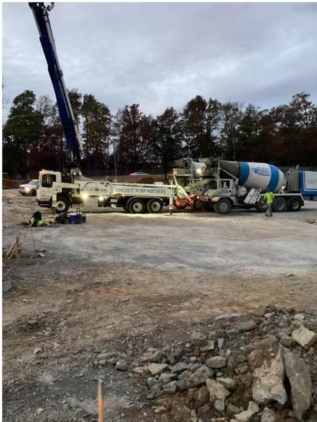
Description: Boom truck setup Image Date Taken: 10/27/2023 Photographer: Miller, Kevin
