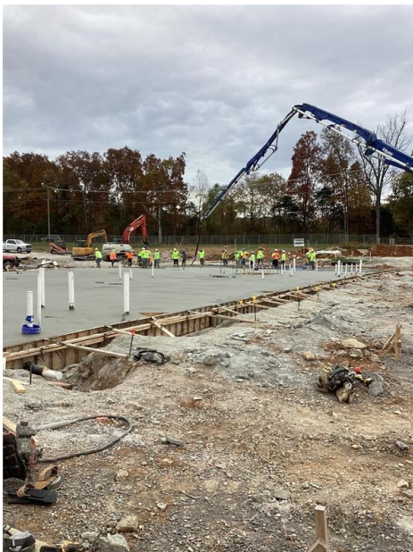
Description: SOG placement Image Date Taken: 10/27/2023 Photographer: Miller, Kevin
