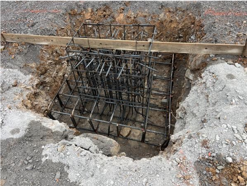
Description: Footing Rebar
