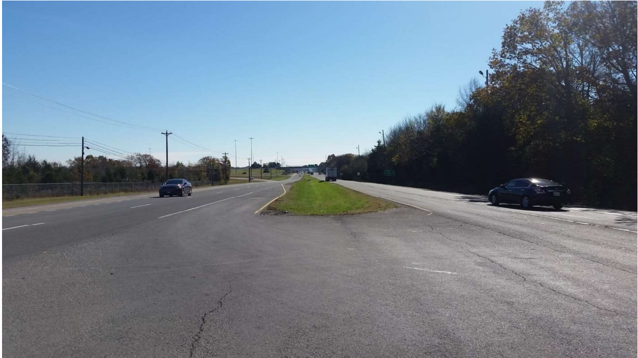
North and Southbound lanes of SR-1 intersection at Jefferson Pike (L.M. 3.45)
