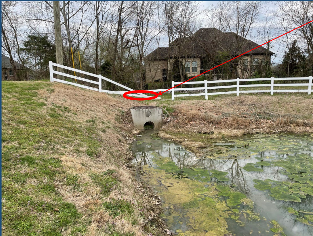
POND OUTFALL STRUCTURE
